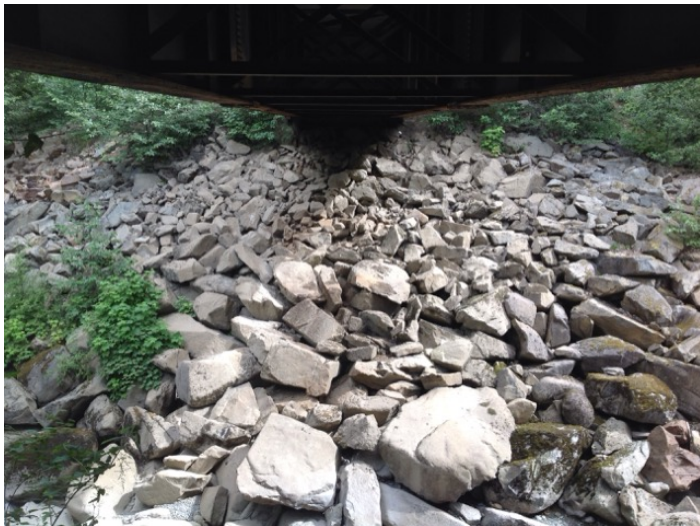
Right Bank Abutment when facing downstream
