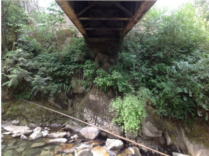
Left Bank Abutment when facing downstream
